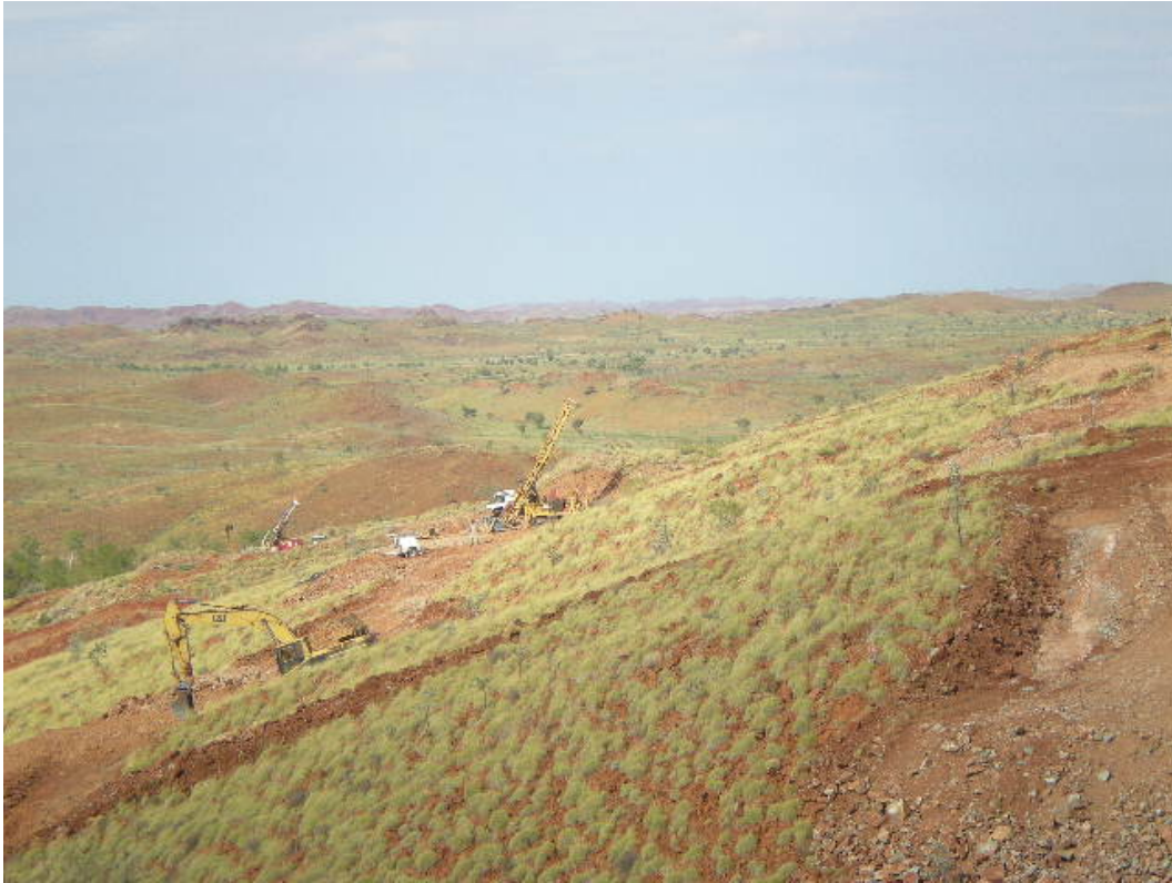
Big Hill Tungsten Deposit Core Drilling Rigs and Excavator in Foreground
