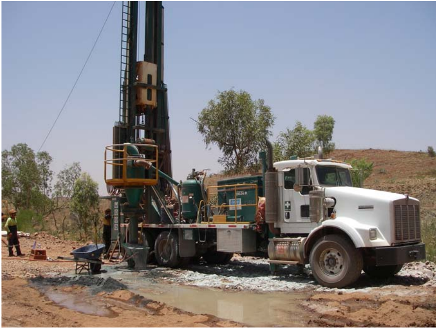
Water exploration drilling
