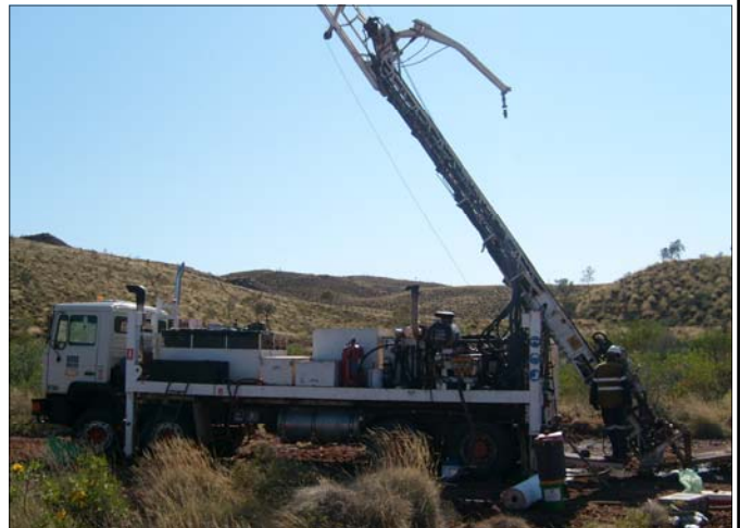
Diamond core drilling at Big Hill - September 2008
